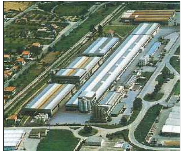
Alfagomma Rubber Industrial Hose Manufacturing facility-Teramo, Italy
